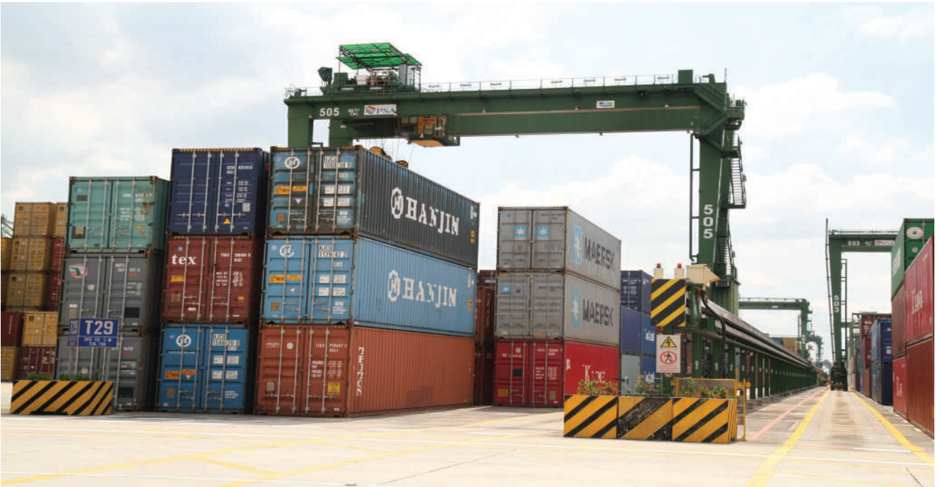
▲ Electric-automated RTG cranes at PPT. PSAC aims to progressively electrify all diesel-based port handling equipment and vehicles at its container terminals.
