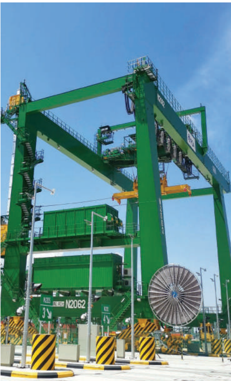
▲ Full electric-automated rail mounted gantry cranes at Tuas Port Phase 1.
